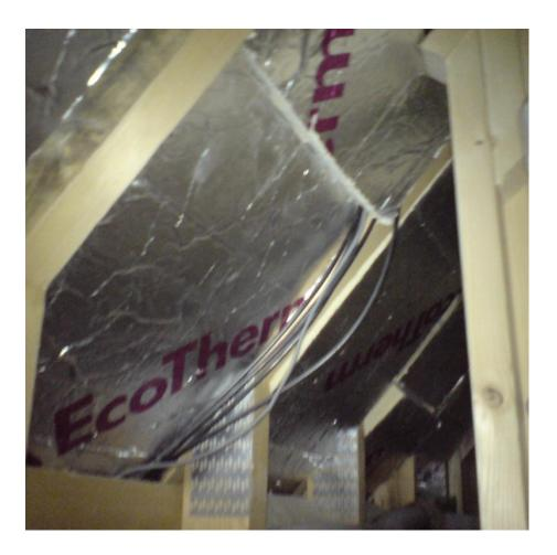
This photograph shows clearly that the insulation has not been fixed in any way within the rafters, some of the insulation can be seen to have moved, none of the joints have been sealed or taped to prevent air flow around them. Cables can be seen threaded through an open joint.
