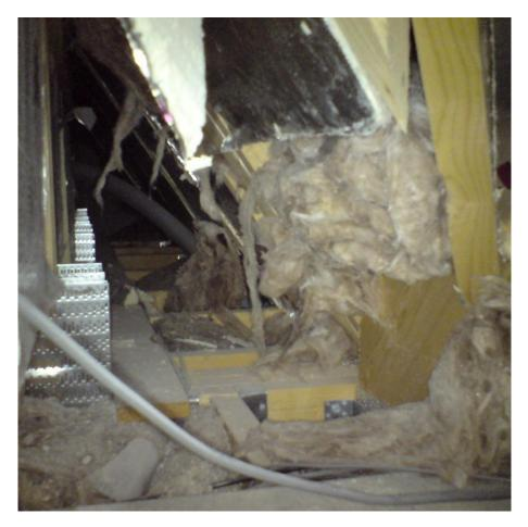
This photograph shows insulation falling out of position, fibre glass insulation has been stuffed into some of the gaps between the solid insulation board, it is poorly installed and likely to fall out over time and looks like a 'bodge job', not what you would expect to see produced by a professional builder.
