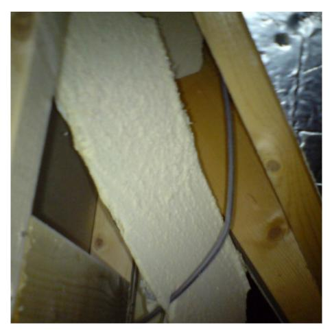
The photograph above shows a piece of the rafter insulation that has actually fallen out of position, it is actually being prevented from fully falling out by an electrical cable which is supporting it! Above this piece of insulation is the underside of the roofing felt allowing free external air to flow into the roof void.
